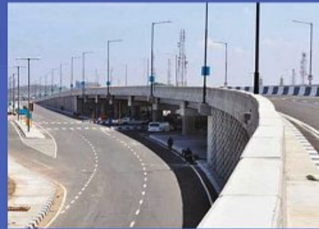
Ajah Jubilee Flyover Bridge (NIGERIA)
